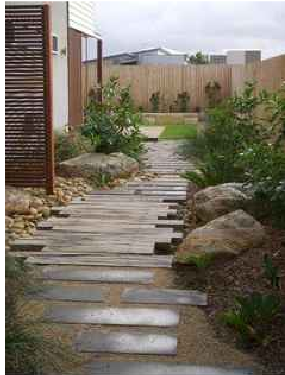
RECTANGULAR PAVERS AND BRIDGE OVER SWALE
